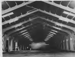
The industrial building is 75 ft. wide and 300 ft. long. E edificio industrial ta 75 pie hanchu y 300 pie largo.
